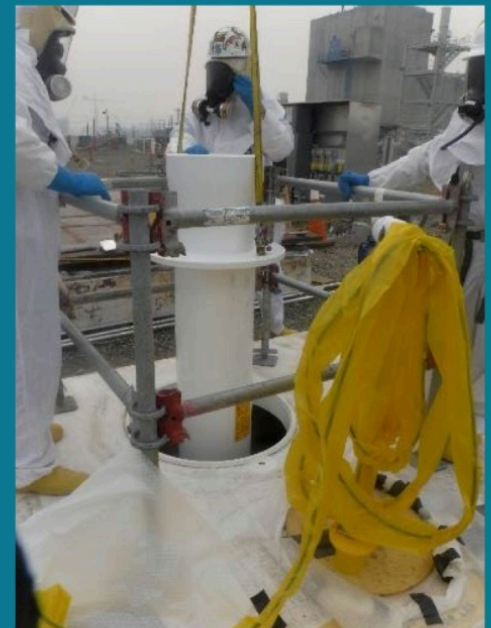
Workers prepare Tank A-101 for future waste-retrieval activities.
