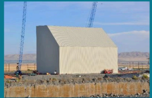
K East Reactor Interim Safe Storage enclosure, completed in October 2022.
