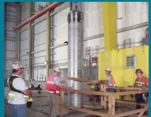
Workers handle an empty multicanister overpack, used to store irradiated spent nuclear reactor fuel.
