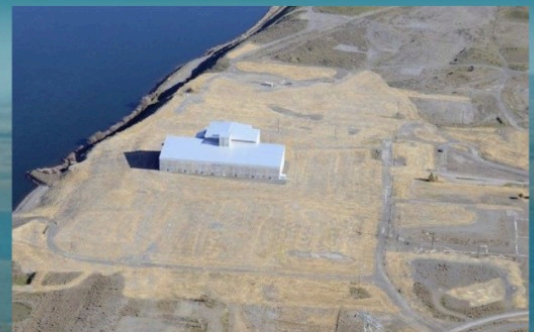
N Reactor in 2015, after Interim Safe Storage.
