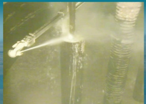
High-pressure water is used to break up waste in Tank AX-101.
