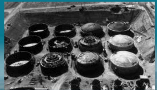
Tank Farms under construction.
