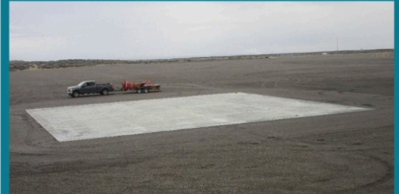
This 80-by-80-foot concrete pad at the Integrated Disposal Facility will be used to stage some waste prior to encasing it in a special cement-like substance.
