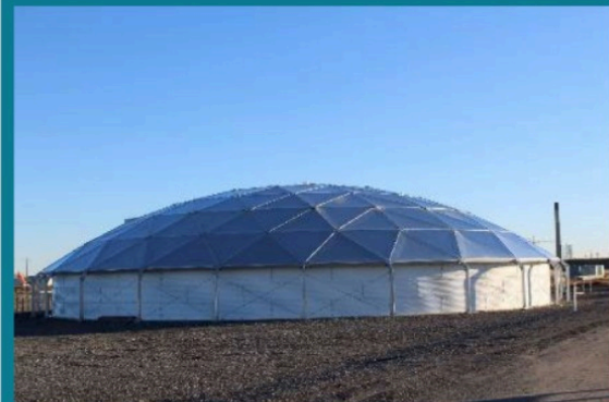
The Integrated Disposal Facility includes two 400,000-gallon tanks to collect potentially contaminated water from rain and dust-suppression activities.
