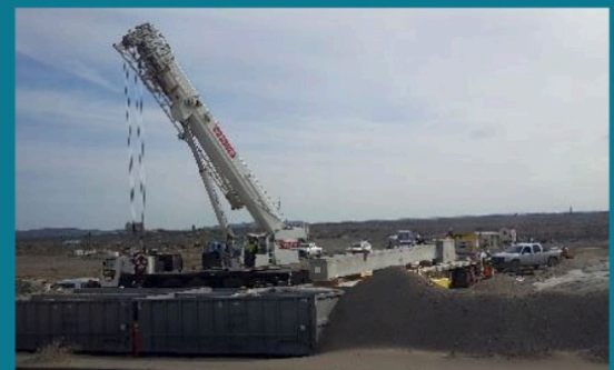
Workers use a crane to place a large item into a Super Cell for disposal.
